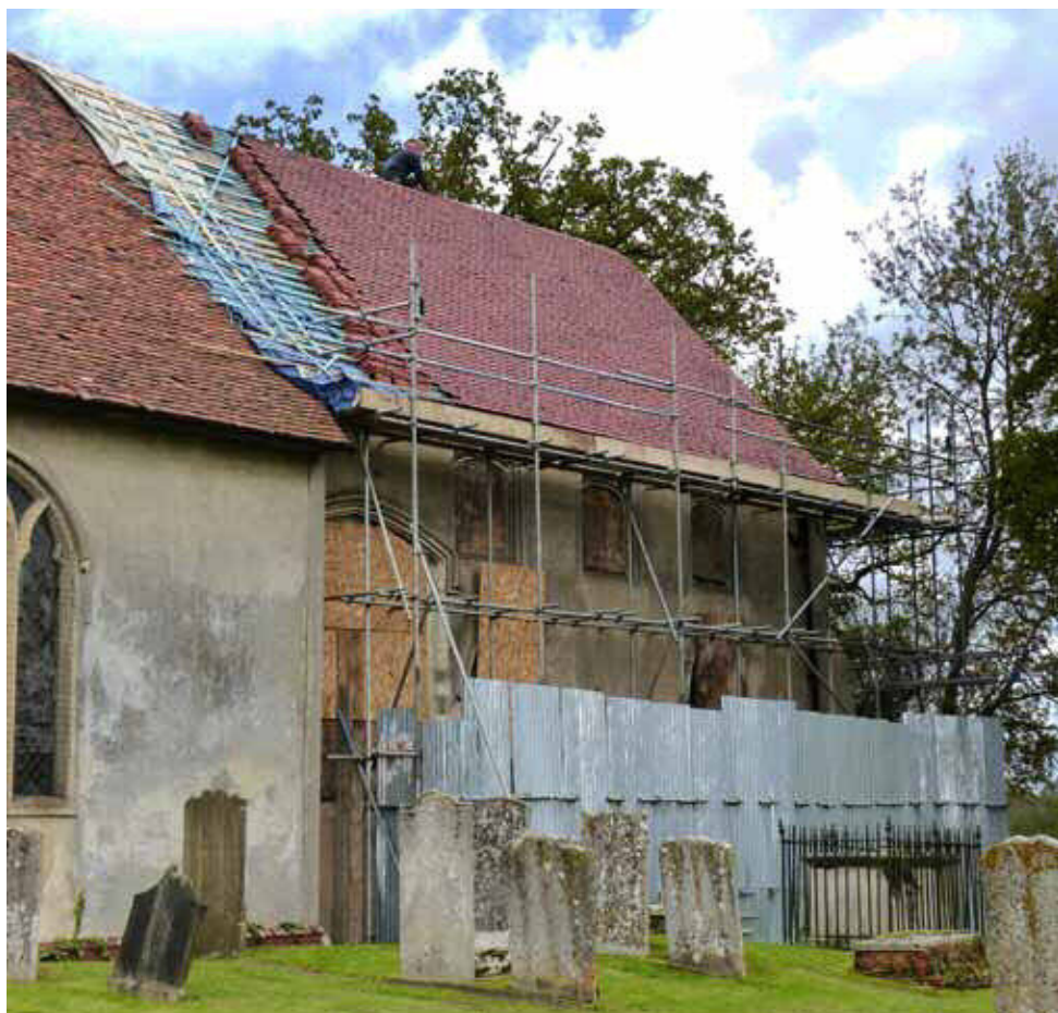
A grant of £15,000 to St Margaret's, Stanford Rivers in 2014 helped to get the church roof re-tiled last year.
