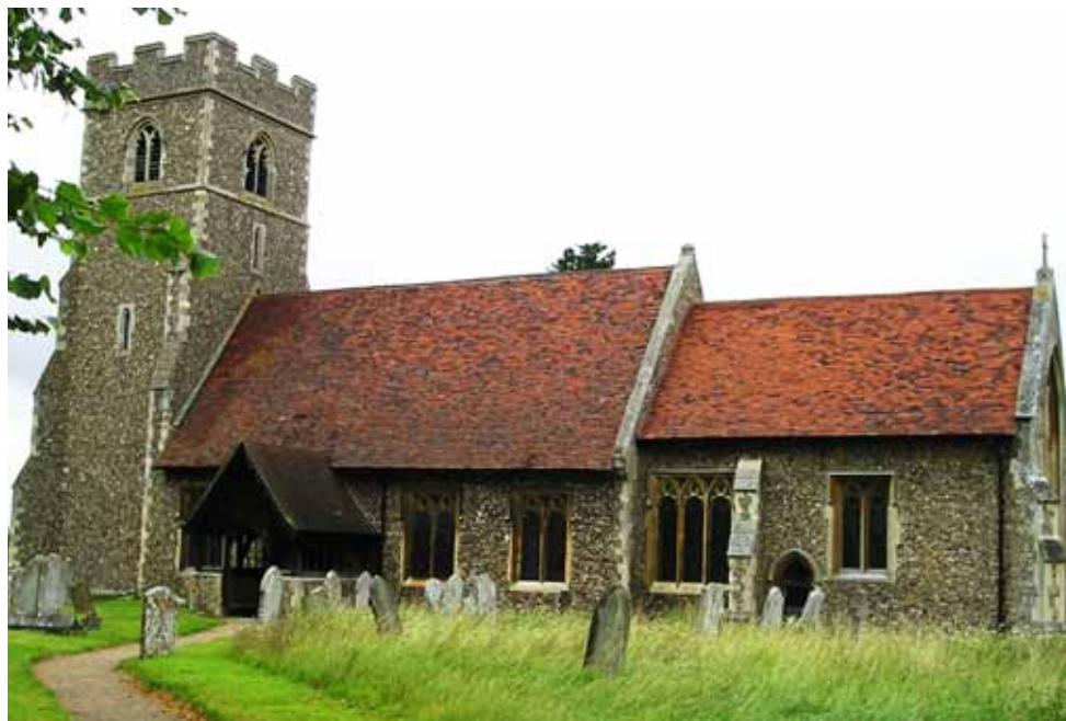
St Christopher's Church in Willingale was awarded £15,000 for roof repairs
